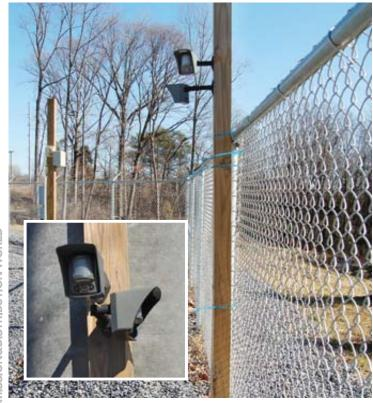
Video monitor installation just requires mounting of the wireless cameras to observe the station fence perimeter.
