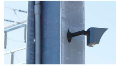
This is a close-up of the video monitor camera located inside the station and "looking" out toward the perimeter fence.
